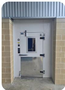
Insulated exterior entrance
